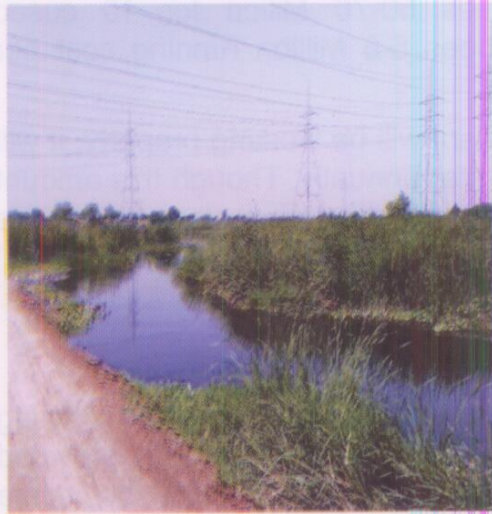
Fig. 5 Drain at Babu Sabu
