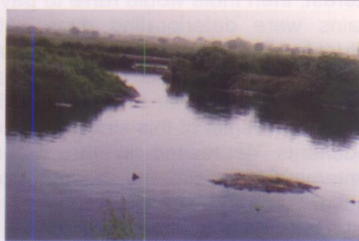
Figure-4: Shalimar Escape Channel discharging wastewater without treatment into River Ravi
